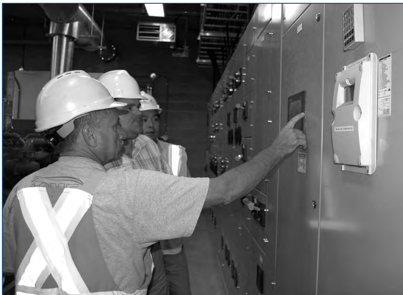
The SUMA policy team had the opportunity to learn the 'ins and outs' of water infrastructure delivery during a tour with the City of Regina. Here, Policy Director Mark Cooper and Policy Analyst Che-Wei Chung are shown the controls for a lift station.
